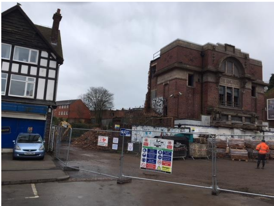
The view from the High Street after the demolition of the auditorium.
