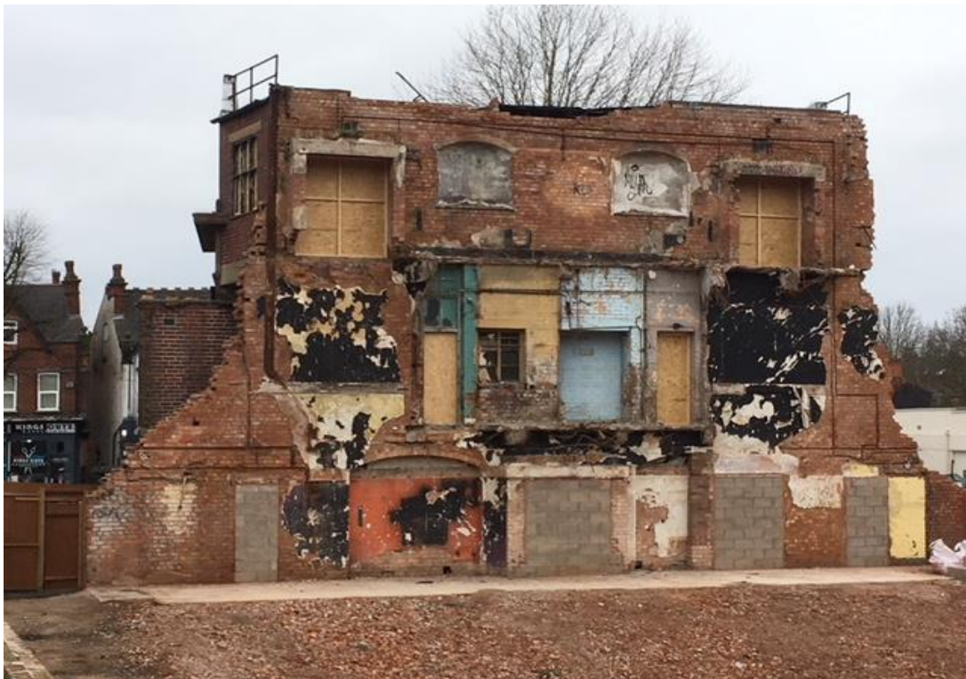
The rear of the foyer block after demolition waiting for the new development to be added to it.
