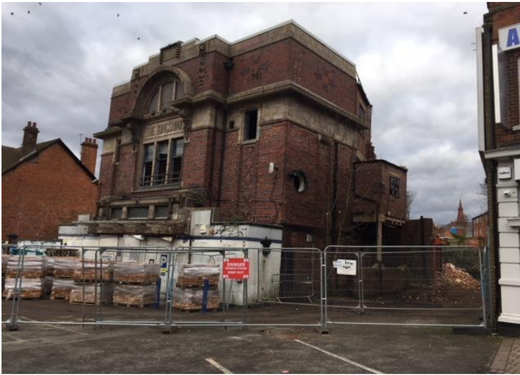
The view from the High Street, old Municipal Bank site, after the demolition of the auditorium.
