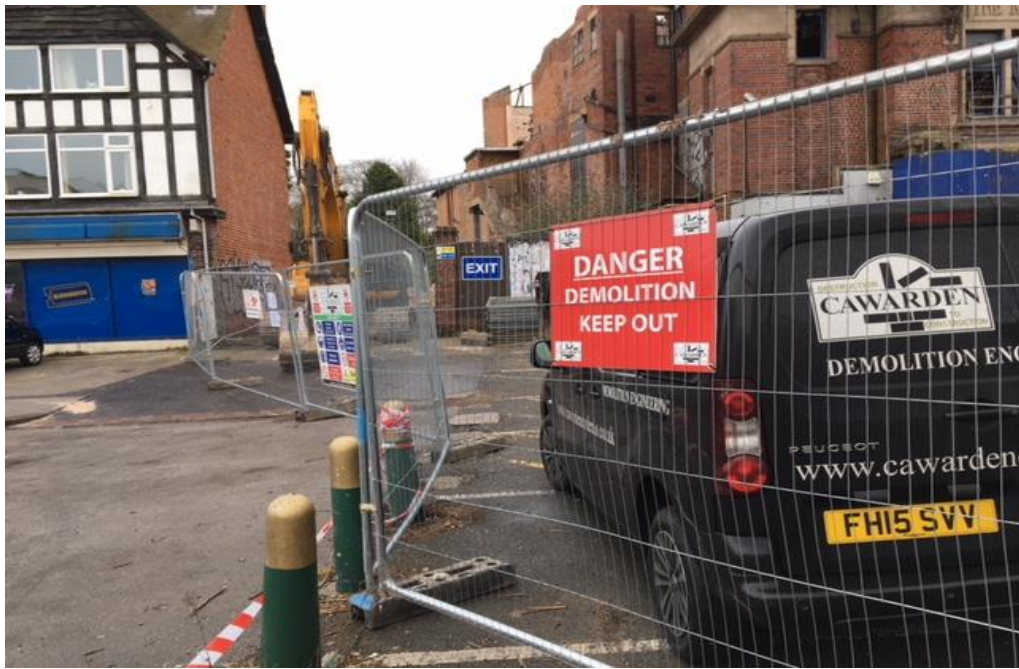
All fenced off and demolition has begun.
