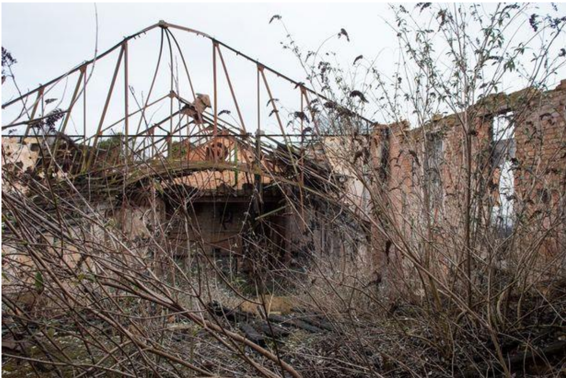
The inside of the auditorium, having been taken over by nature, before demolition started in 2018.
